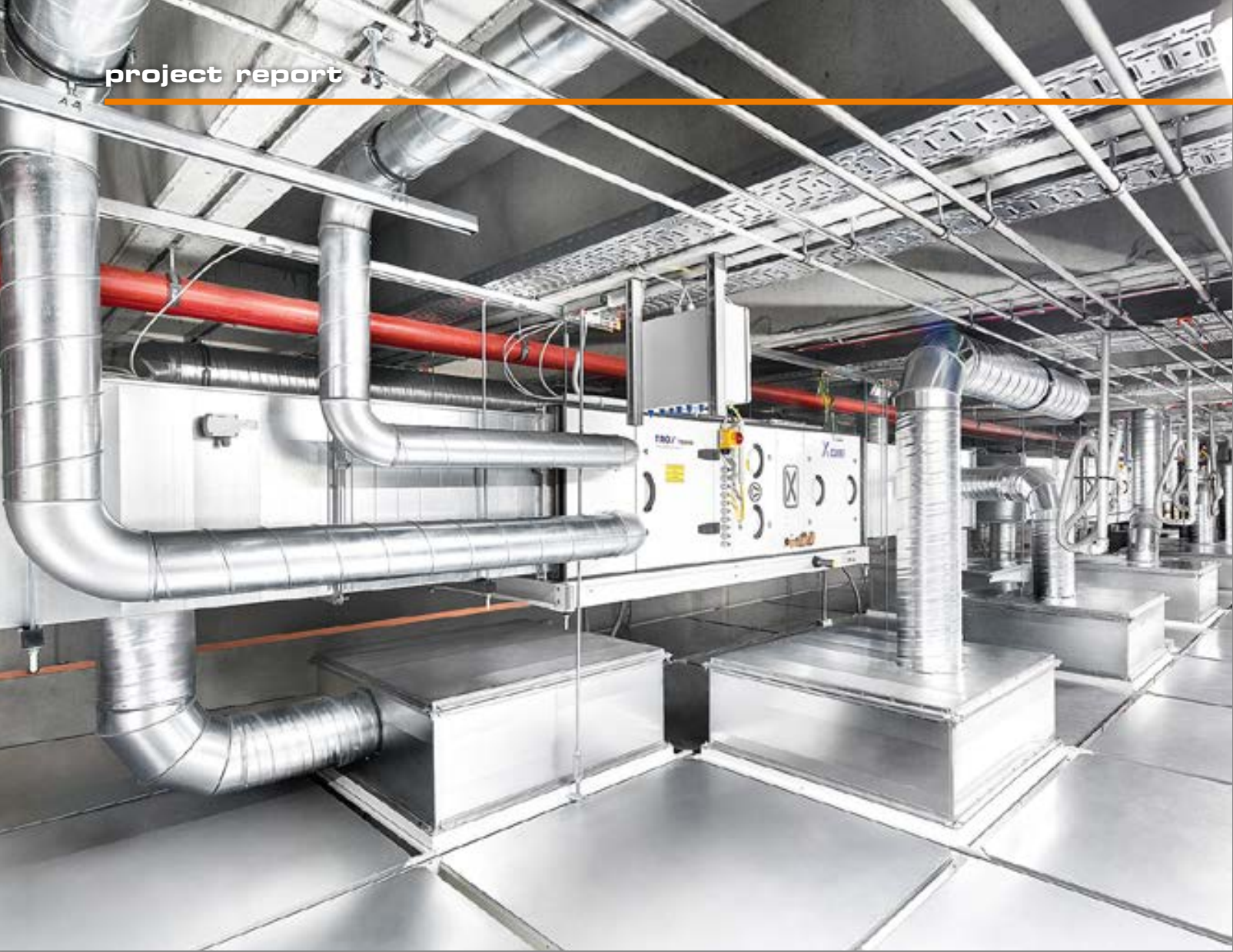
The X-CUBE CROFCU (Clean Room Fan Coil Unit) ventilation system is a particularly economical solution for clean rooms.
